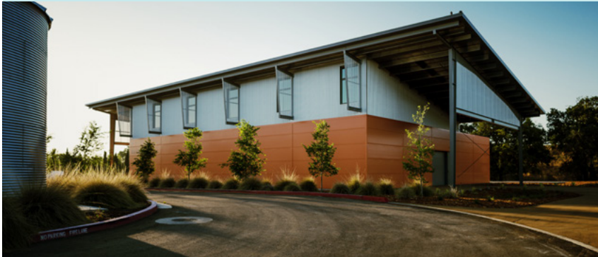
FIGURE 4.7: JESS S. JACKSON SUSTAINABLE WINERY BUILDING AT THE UNIVERSITY OF CALIFORNIA AT DAVIS CAMPUS.
