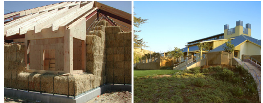
Source: Camp Arroyo, Livermore, CA. Dining Hall. Straw bale construction. Photos courtesy of Siegel & Strain Architects and JD Peterson.
