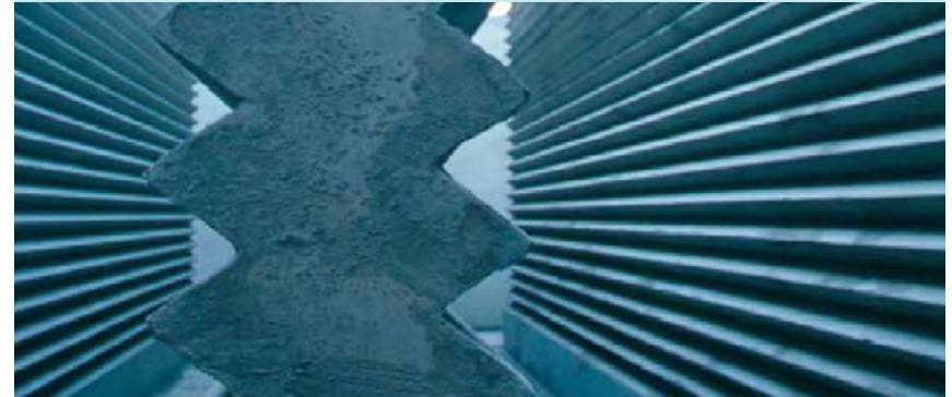
FIGURE 4.8: A SECTION OF THE 1.4 KILOMETER THERMAL LABYRINTH THAT RUNS BELOW FEDERATION SQUARE IN MELBOURNE, AUSTRALIA.
